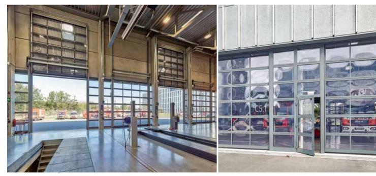
The doors travel up as a complete element and therefore leave space under the ceiling for supply lines.
