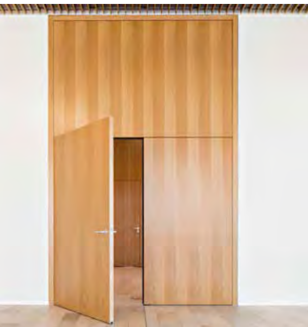
The doors appear to be room-high thanks to transom panels. The clear passage width of the fire-rated and smoke-tight door can be extended if necessary.
