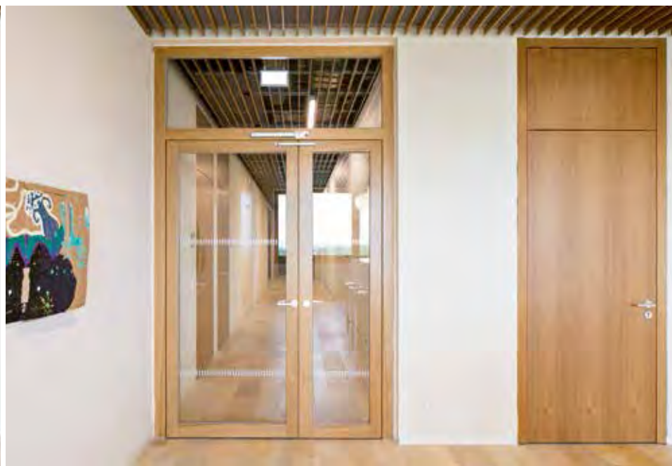
The doors appear to be room-high thanks to transom panels. The clear passage width of the fire-rated and smoke-tight door can be extended if necessary.
