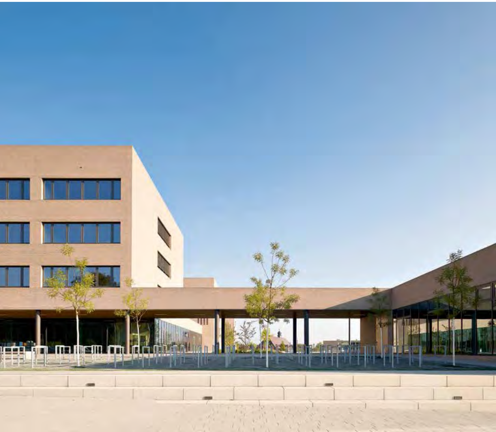
The entire building is homogenously covered by a grey beige brick facade made from hand-painted special-format stones.
